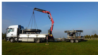
12ton hiab truck and trailers
